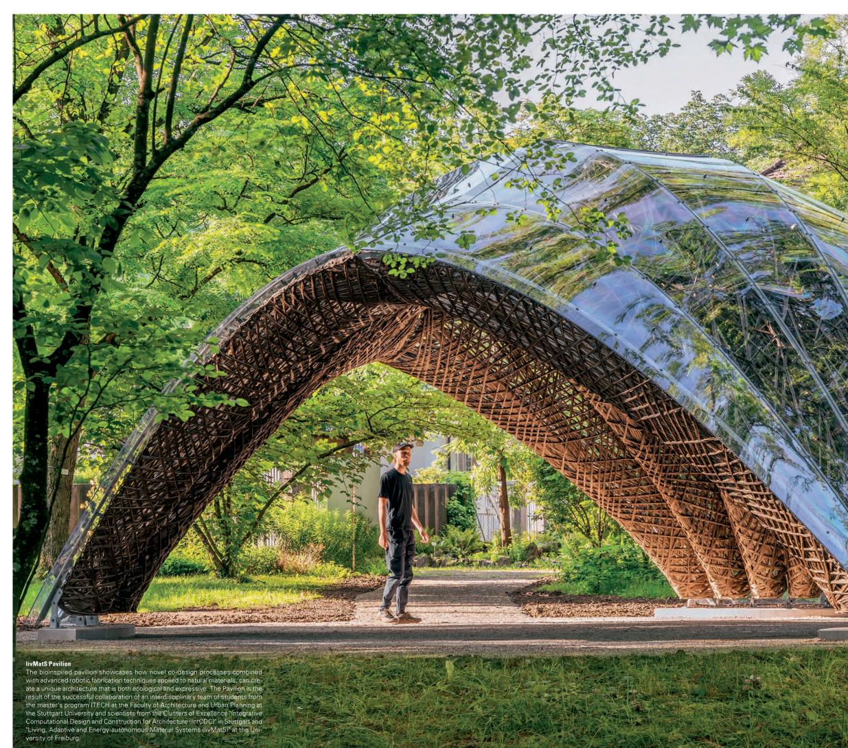
The structural components of the pavilion are robotically wound in a coreless fila-ment winding process using flax fibers, a natural, biodegradable material which is regionally available in Central Europe. The natural fibers and their biological variability presented the researchers with new challenges.
